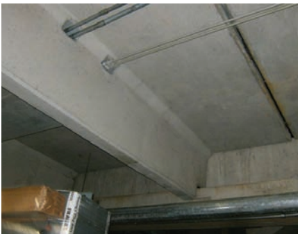
Post-tensioning standard conduit pass through double tee stem blockout.
