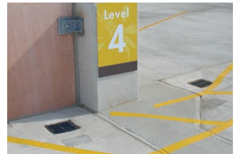
Cast-in drains are positioned at the corners of double tees.
