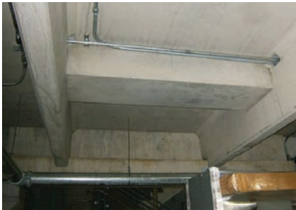
Precast stressing bulkhead resists post-tensioning forces.
