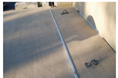
The TeeCurb System directs stormwater to drain without expensive concrete curbs, ski slopes, or pour strips.
